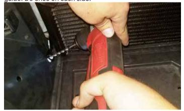
15. Secure the lower portion of the LTR to the air ducts using two (2) M6 x 16mm bolts and two (2) M6 locknuts from hardware Bag #2.
